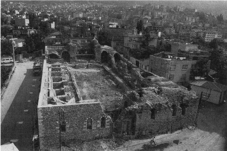
Figure 4.16. Bursa, I. Yildirim Beyazit Darüssifasi, with timbers cut in 1400. Cubicles for the patients are ranged left and right. The foundations of the interior arcade carried pipes for running water. (P. I. Kuniholm, ADP)
